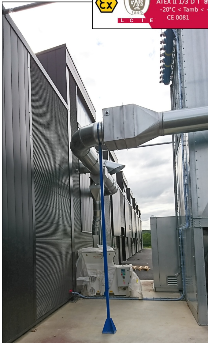
Clapet anti-retour CATA Ø 600 mm
